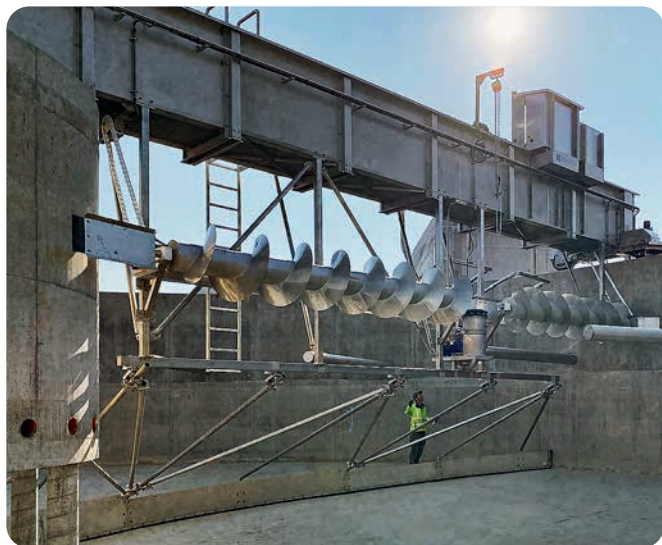
Circular scraper with floating sludge extraction system
