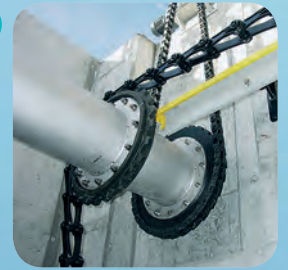
Stainless steel/GRP main shafts
