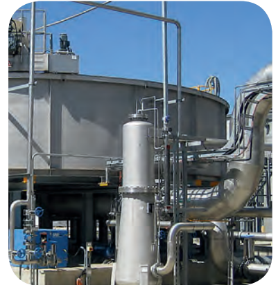
High-performance saturation system for the production and insertion of micro-bubbles in the flotation tanks
